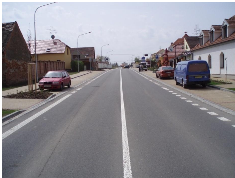
Fig. 3. Road II/422-Lednice – after the implementation
